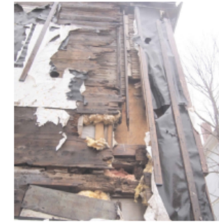
PHOTO - EAST - WATER DAMAGE SCALE: 1/4" = 1'-0"
